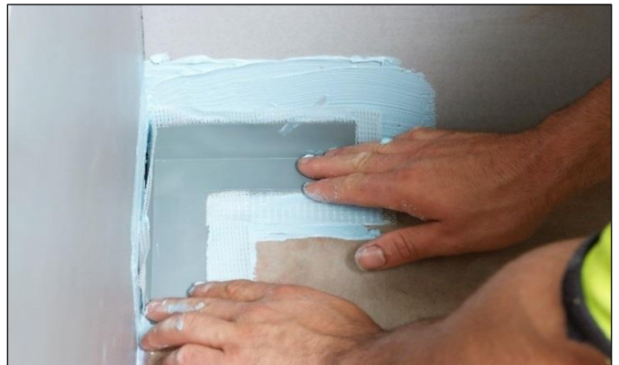
Installing Elastoproof Prefabricated Corners
